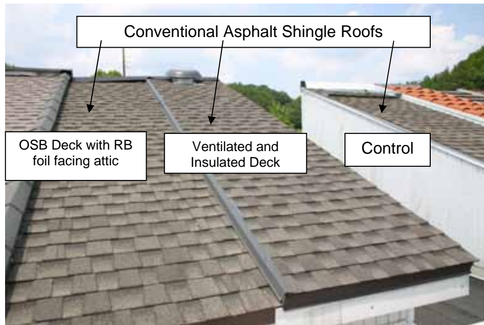
Figure 2. Envelope Systems Research Apparatus (ESRA) with the rightmost roof lane identified as the control system (conventional asphalt shingle roof system), the ventilated and insulated roof deck (center lane) and conventional roof system with foil-faced OSB deck (far left lane).
